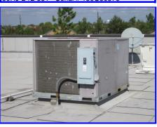
Unit 2 is a Carrier 7.5 ton unit - Model # 50HJ-008-521 - Serial # 1300G30234
