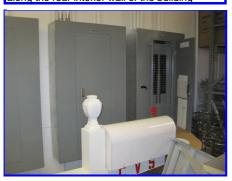
The main electrical panels should be free of clutter 3 feet in front of the panel service doors
