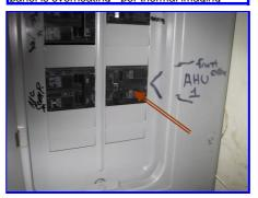
The 30 and 40 amp breakers in the sub-panel are overheating per thermal imaging
