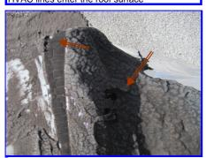
Repair loose electrical conduit at unit 2 in the center of the roof - left center unit
