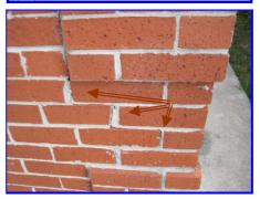
Repair loose brick mortar along the rear wall exterior corners on both sides of the rear door
