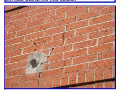
Also the bathroom exhaust vent on the left side wall is missing an exterior cover
