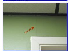
There are settlement stress cracks above the right side middle office door at the header
