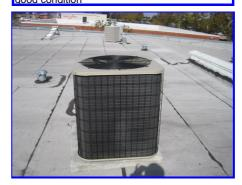
Reseal HVAC cover of unit 3 where HVAC coolant lines enter the roof cover
