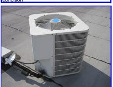
Reseal open seams in the tar seal of unit 4 where the HVAC lines enter the roof covering
