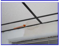
Water stain in rear left room ceiling - possible HVAC condensation or old roof leak
