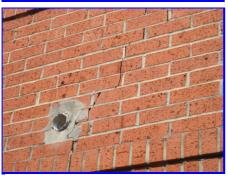
Settlement cracks at the left side wall are greater as the settlement travels up the wall
