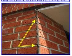
Seal around the exterior wall at the concrete pad that circles the building to prevent water penetration
