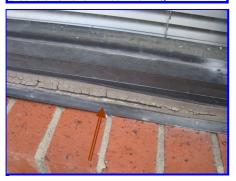
There are horizontal cracks along the right side wall at the mid-section
