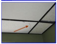
There is stress cracks present above the rear right hallway door
