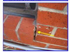
Replace all bridle and cracked window sealant around all exterior window framing
