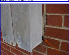
Repair loose conduit at the rear wall and seal around the openings
