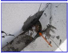
All seals on the upper cap of the knee walls around the roof should be coated with tar sealant
