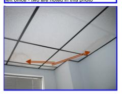
3rd Water stains in rear left room ceiling near left exterior wall
