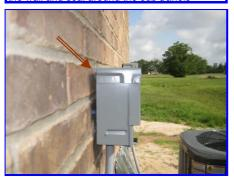
Seal around the HVAC covers where the lines enter the side wall
