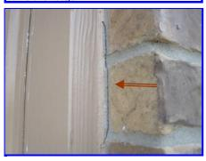
Seal around and re-paint the surface of the front roof vent
