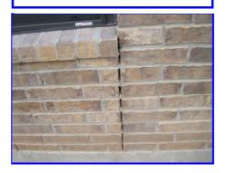
Seal all exterior wall inside corner seams of the brick veneer
