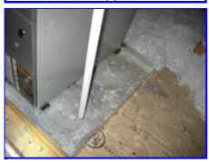
Insulation in hot water heater drip pans
