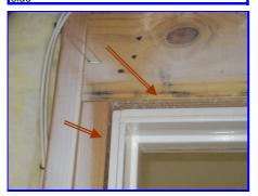
Repair loose insulation along the game room rear wall in the attic
