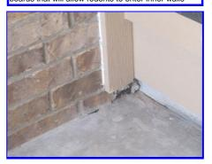
Correct erosion at front sidewalk - recommend French drain on inside portion
