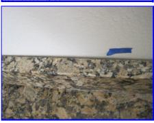
The far right corner of the master tub is cracked
