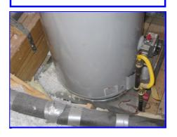
The top of all evaporator plenums are not properly sealed at the upper seams
