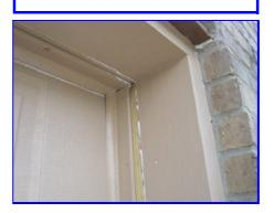
Seal gaps around the exterior garage door trim at the brick edge
