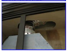
The exhaust fan cover is not installed
