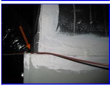
The rear furnace exhaust vent is disconnected and laying on the attic deck
