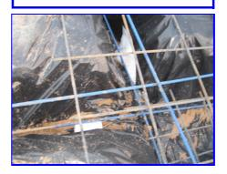
Vertical rebar supports should be on the inside of the form for the cable they are supporting
