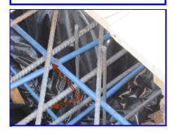
Several post-tension chairs are improperly placed or damaged
