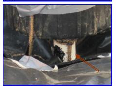
Slab thickness measures 3.25 inches at center rear area of the form
