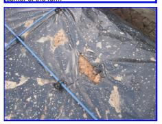
Vertical rebar supports should be on the inside of the form post-tension they are supporting
