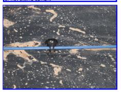
Water is standing in some of the footing trenches (Beams)
