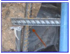
Damaged chairs are allowing cables to lie on top of the form
