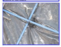
More photos of rebar ties missing at repair junctions
