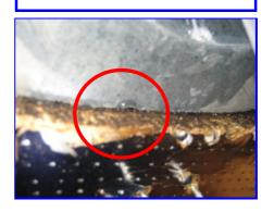
Abnormal gaps have already formed in the sealant of the side wall expansion joints
