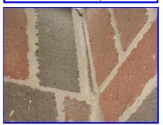
Settlement cracks in the brick mortar at the base of the front door - both sides
