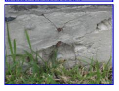
Settlement gaps have already formed at the abse of the rear door brick mortar
