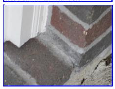
Significant chip in front porch slab - left of front door
