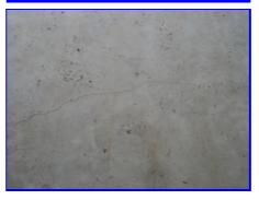
Several settlement cracks in the garage slab radiating toward the home's slab
