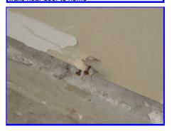
The front right side walk has been crushed from direct weight application
