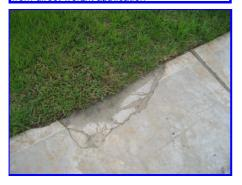
Significant settlement cracks in the garage slab that radiate across the garage floor
