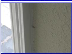
The wall beneath the kitchen bar is severely bowed at the base
