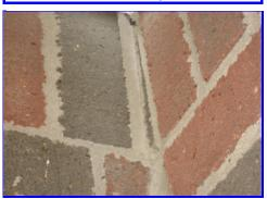
Settlement cracks in the brick mortar at the base of the front door - both sides
