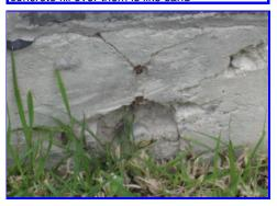
Settlement gaps have already formed at the abse of the rear door brick mortar
