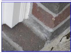
Significant chip in front porch slab - left of front door
