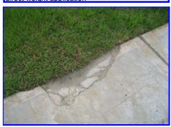
Significant settlement cracks in the garage slab that radiate across the garage floor
