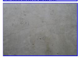
Several settlement cracks in the garage slab radiating toward the home's slab
