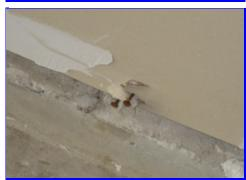
The front right side walk has been crushed from direct weight application
