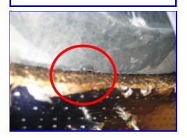
Abnormal gaps have already formed in the sealant of the side wall expansion joints
